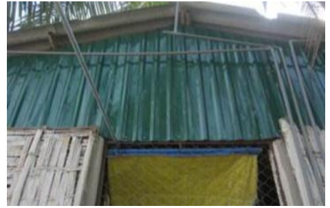
The water cooling system is made from locally available pipes and hoses, and automated with simple pumps and timers.
