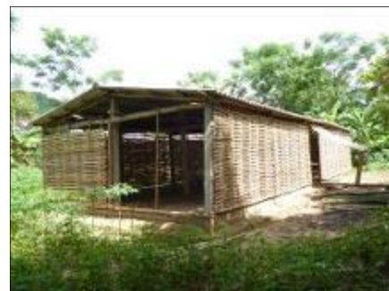
The completed communal grow house in Dakrong
