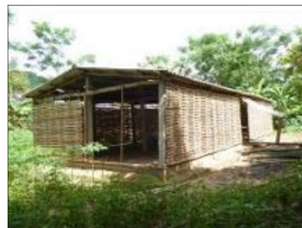
The completed communal grow house in Dakrong
