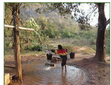
A villager uses the new gravity fed water system in Kaengyalouan Village
