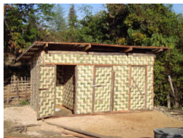
Latrine block in Phonkham village
